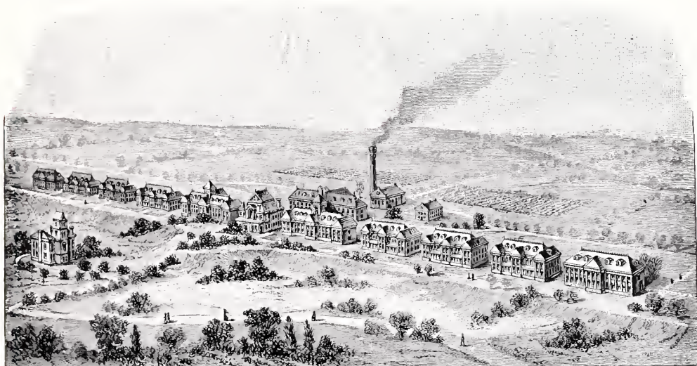
Northern Hospital for the Insane, Logansport, Ind., with 400 H. P. of Babcock & Wilcox Boilers. Erected 1885.
